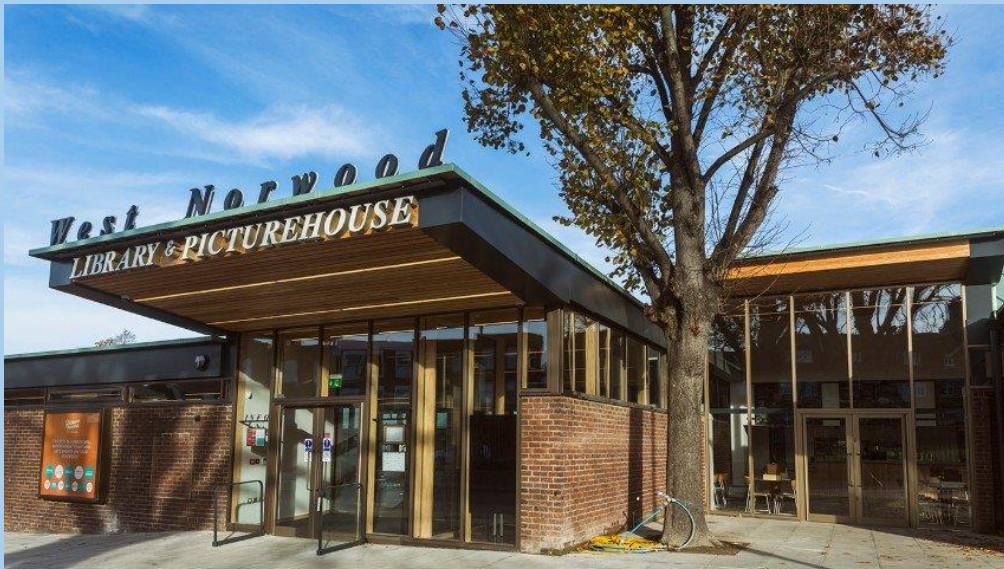
West Norwood Library and Picturehouse
